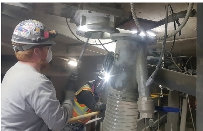
Removing hardened cement chunks from the silo gate to re-establish material flow.
