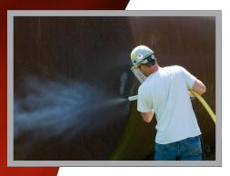
Media blasting is an all-encompassing term used to describe a wide variety of abrasive blasting. Commonly referred to as sandblasting in the past, media blasting has become the preferred term as it can refer to any type of abrasive blasting or dry ice blasting. Because using sand can carry serious health hazards, many types of other materials are used today with soda blasting the most common.
