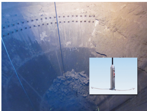
Exposed silo cone after cleanout started with JR360H.
