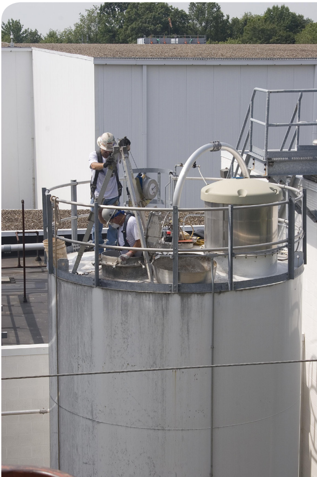
Figure 2. Typical rigging for a small opening and one engineer.
